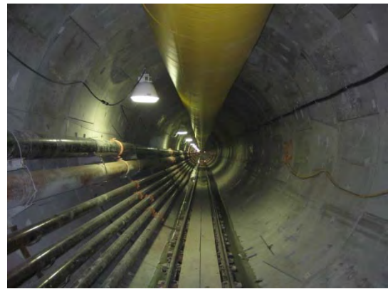
Figure 3-6 (left) Stacked Precast Concrete Segments and Figure 3-7 (right) The Assembled Ring in the Tunnel with Lighting, Yellow Ventilation, Utility Pipes and Railroad Tracks in the Tunnel during Construction
