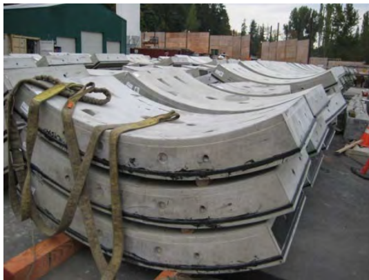
Figure 3-6 (left) Stacked Precast Concrete Segments and Figure 3-7 (right) The Assembled Ring in the Tunnel with Lighting, Yellow Ventilation, Utility Pipes and Railroad Tracks in the Tunnel during Construction
