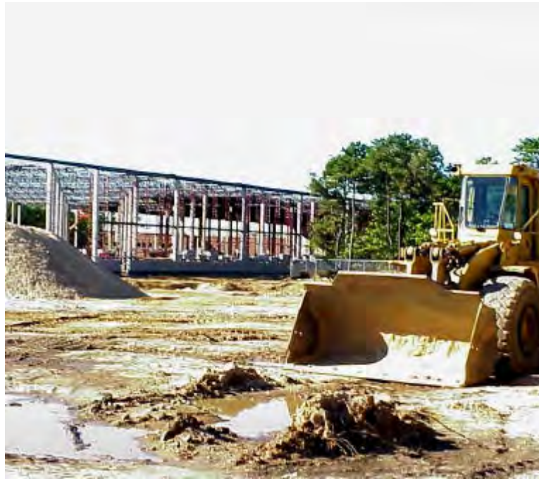
Figure 26 Industrial project under construction on Veterans Memorial Highway, Bohemia - October 2000.
