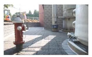
went with permeable pavers. The pavers are set on top of a layer of sand. The rainwater is able to seep back into the ground. The project was completed in the beginning of 2010. To date there have been no problems with flooding.
