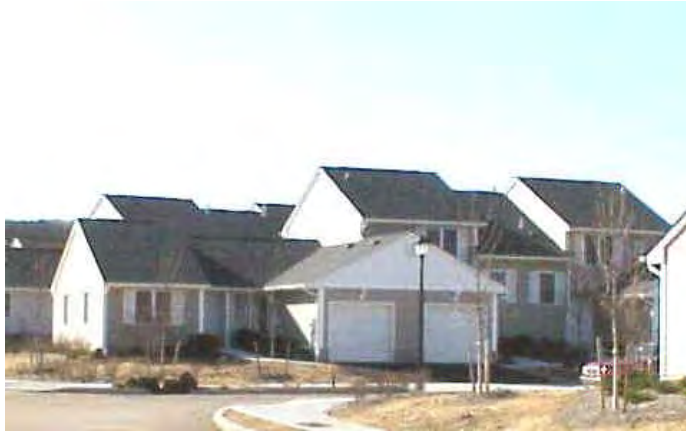
Millennium Hills is a 44 unit affordable housing development in Melville, under construction in 2003.
