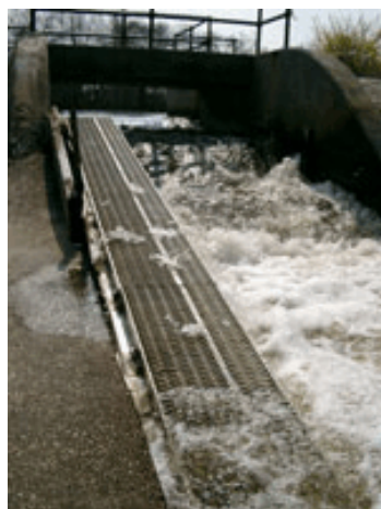
The Grangebel Park fish ladder allows diadromous fish to travel up the Peconic River to spawn.
