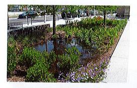
Rain gardens reduce stormwater runoff volume by temporarily storing water and returning it to the ground, reducing the immediate volume load on water bodies and the storm drain system by up to 98% which in turn helps to reduce the risk of flash floods (Upstate Forever). In 2008, the Saylors Grove bioretention basin intercepted 73% (25.4 of 34.8 million gallons) of stormwater runoff and resulted in a significant reduction in rainfall intensity peak flow (Howley).
